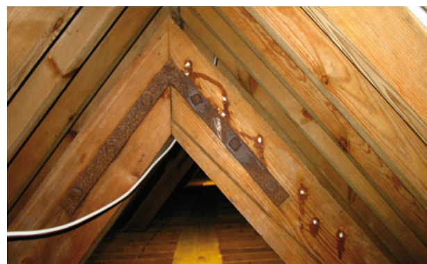
The rods were then cut flush with the timber surface
