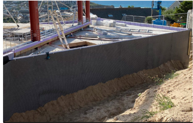
Installed ICF blocks protected by Triton Double Drain.
