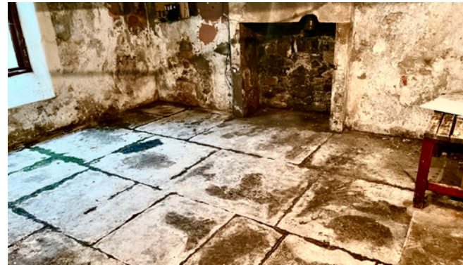
The basement prior to conversion
