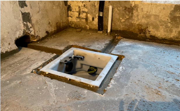
New XL sump set in floor
