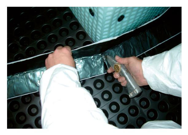
Fig. 12 Cornerstrip pressed into position
