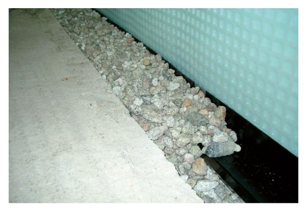
Fig. 22 AquaChannel installation including inspection port
