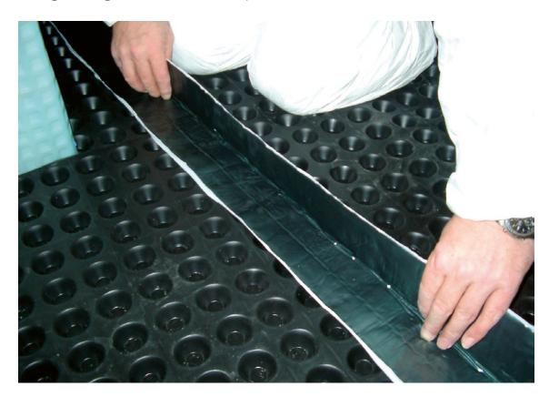
Fig. 9 Forming  $90^{\circ}$  angle crease in Cornerstrip
