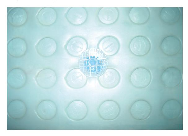
Fig. 17 Fixing Plaster Base Plug between 4 membrane studs
