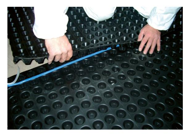
Fig. 7 Positioning membrane stud to stud over Sealing Rope seal
