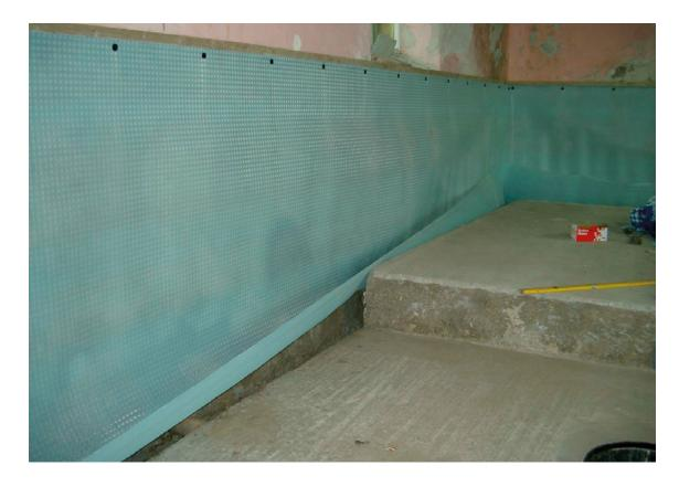
Fig. 20 AquaChannel installed to cast gully
