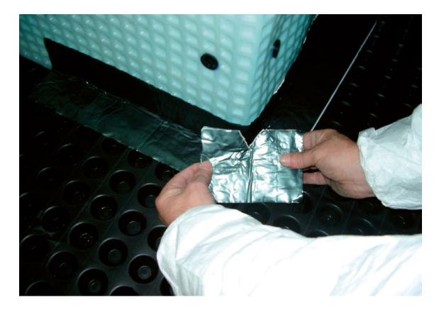
Figs. 13 and 14 Angle piece to seal and complete corner joint
