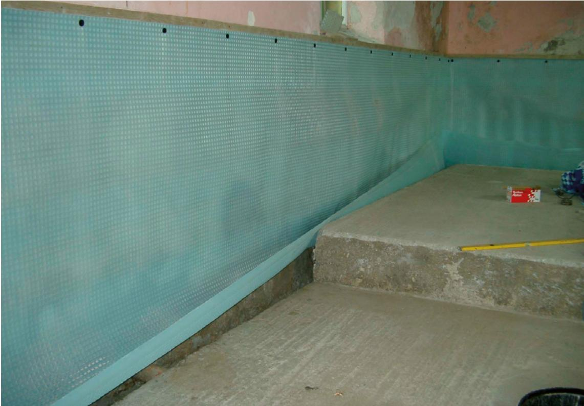
Fig. 20 AquaChannel installed to cast gully
