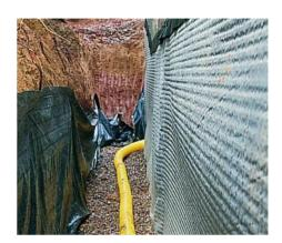
**Platon DOUBLE DRAIN** must be installed over a primary membrane, such as Triton EX100 adhesive sheet membrane, Triton TT Vapour Membrane or, when used horizontally, Triton TWS-Fastcoat. Fix **Platon DOUBLE DRAIN** along the top edge above the primary membrane, with **Platon DOUBLE DRAIN** X-cramps at 250mm centres. Overlap vertical joints by 120mm and horizontal joints by 120mm. Filter fabric can be pulled back for successive overlaps of the membrane.
