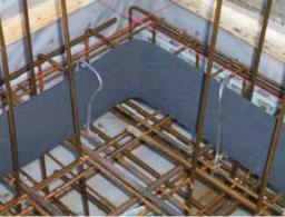
Installation of Triton CEMflex VB Plate Waterstop into the fresh the concrete.
