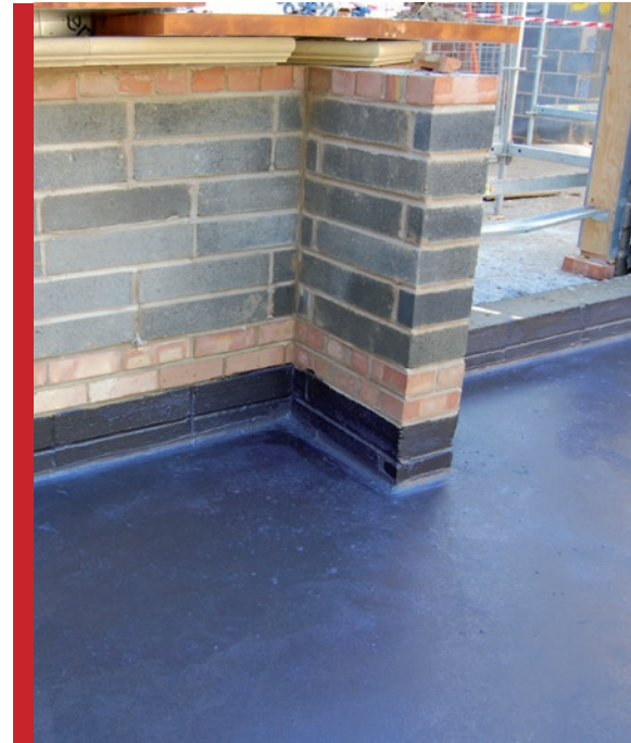
TTVM used as primary waterproofing layer on external basement roof
