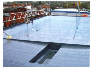
The technically difficult waterproofing of a flat roof can be achieved with a liquid applied system
