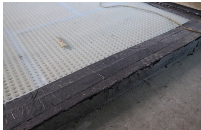
Banded wall to service trench edge detail.
