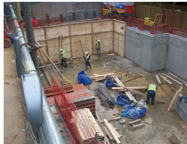
Watertight concrete basement in construction
