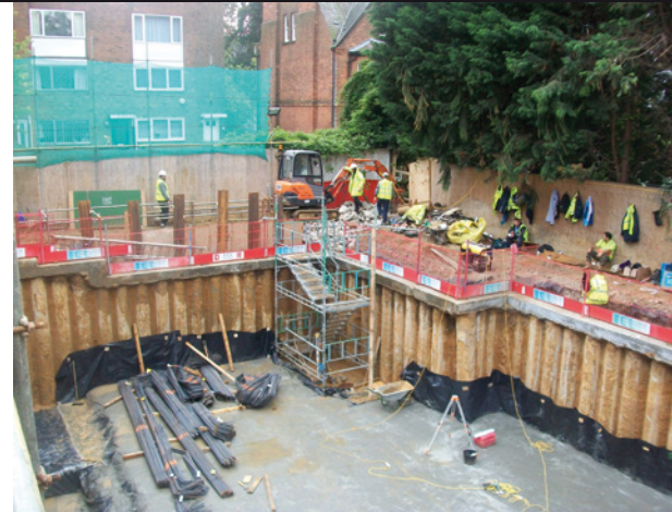
After application of 50mm blinding concrete layer
