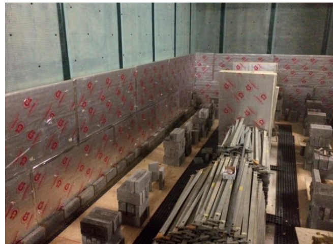
Block wall being installed over insulation and Platon P8 membrane
