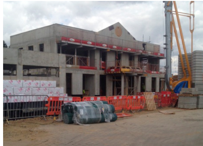
The new concrete frame construction
