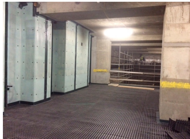
Platon P8 to walls Platon P20 to floor with Corner Strip to seal wall floor junction
