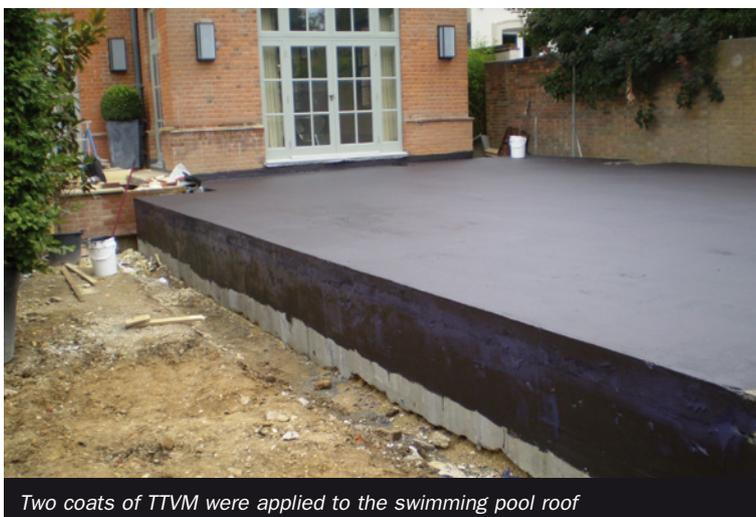
Two coats of TTVM were applied to the swimming pool roof
