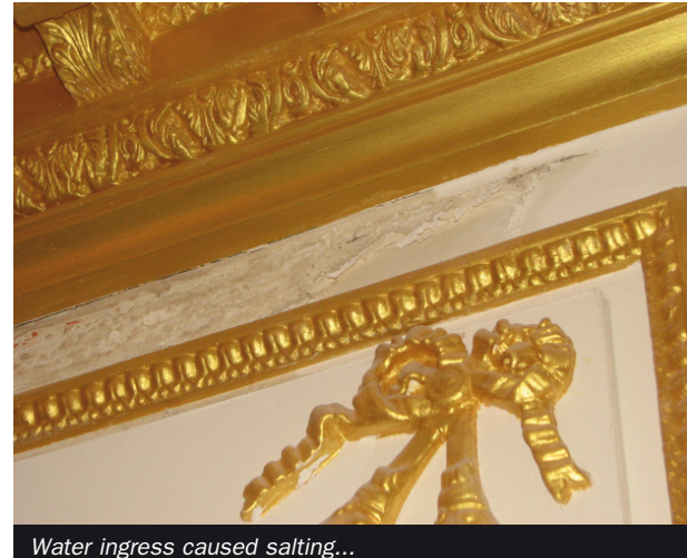
Water ingress caused salting...
