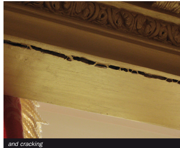
Water ingress caused salting...
