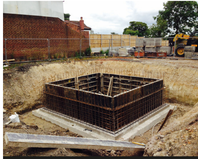
Basement formwork
