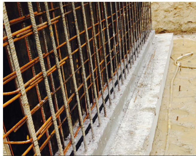
Construction joints waterproofed with TT Waterstop
