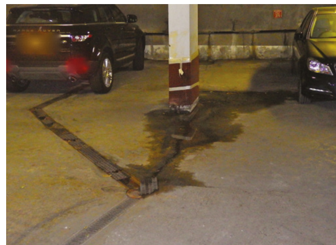
Car park before upgrade
