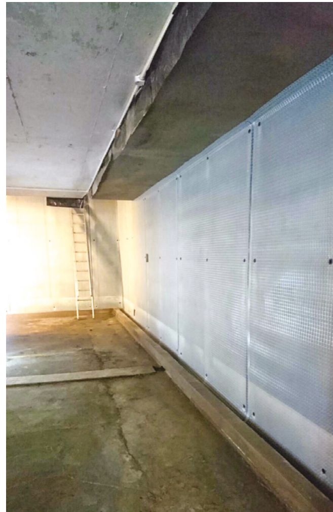
Triton TT55 detail to soffit linked in behind Platon P8 membrane for water to drain down into gulley, prior to installation of Aqua Channel and sealing upstand with TT55
