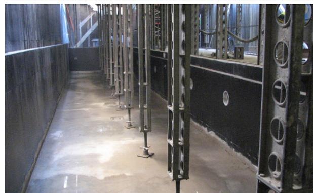
*The concrete walls and floor of the swimming pool were waterproofed with TT Vapour Membrane before tiling*
