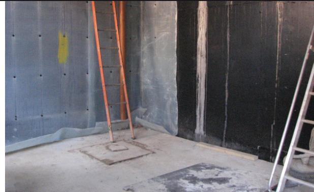
*Cavity drain membranes were installed on the concrete walls after the application of two coats of TT Vapour Membrane*
