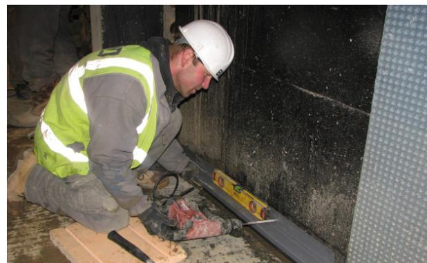
*Checking the fall of the Triton Aquachannel, installed around the perimeter walls, to divert any water from behind the membrane system to the discharge points*
