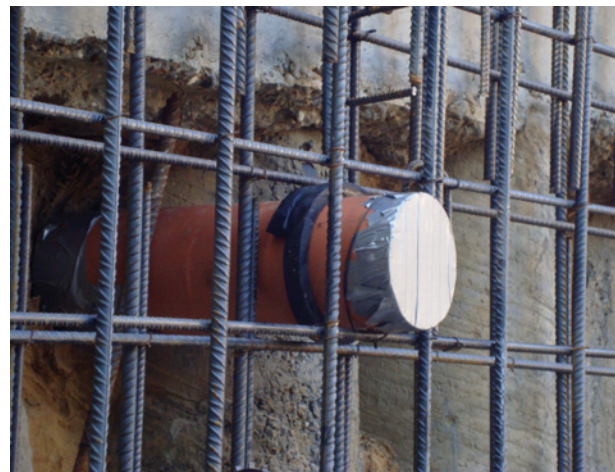
Service entry sealed with TT Waterstop
